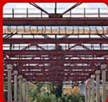
Metal Structure Factory
